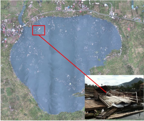
Fig. 11. Aerial image of Lake Palakpakin taken July 2014 after Typhoon Rammasun. It damaged houses, fish cages and destroyed trees. Inset photo is a fish cage with hut damaged by the typhoon.
